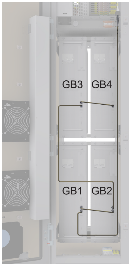
Figure 4.25 Battery communication cables
